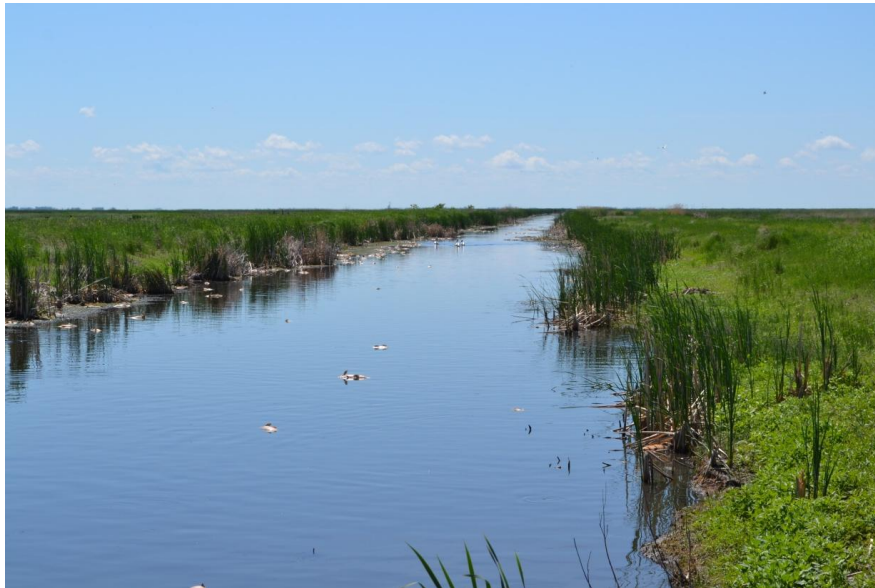
Fig 5. Looking upstream from the gated screens, note some dead carp on the surface in the middle and along the sides of the channel.
